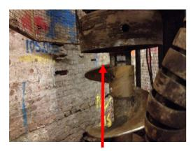
Hand resting on the top flight as duplex lowered onto the next auger
