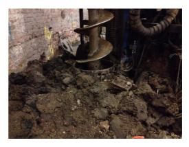
Buildup of spoil leading to uneven ground conditions
