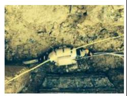
During the installation of the original chamber, concrete had been placed around the WPD LV cable. The CAT signal of the yellow (faded orange)Traffic Signal cable masked the presence of the LV cable cast in concrete below and subsequently led to the incident.
