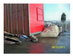
**Photo shows:** Site cabin blown off from lower cabin and resting on 'bean bag safety cushion' at the south-east corner. The site cabin was lifted up by the Contractor's site plant and temporarily propped at the south-west corner. (See over page)
