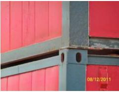
**Photo shows:** View of remaining cabins immediately after incident – cabins are not physically connected or secured to the ground.
