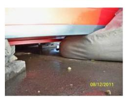
**Photo shows:** View at south-east corner: Site cabin landed on "bean bag safety cushion" and provided approximately 400mm void between the base of the site cabin and the ground level. We understand that the injured party was under the site cabin at this location.
