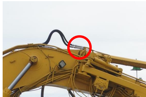
Burst protection repair to dipper ram
