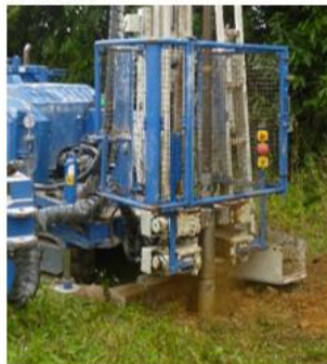
Due to machine setup, guard starts more than 500mm from floor. Either adjust setup or extend the guard.
