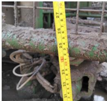
Guard starts more than 500mm from the floor. Must be extended.
