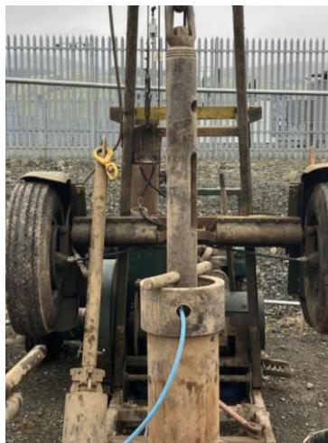
Rig set up
