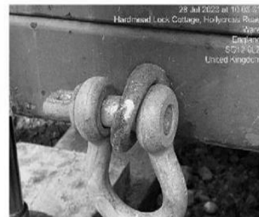
Bow shackle attached to the Lifting eyebolt
