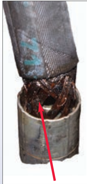
Hose pulled out of ferrule
