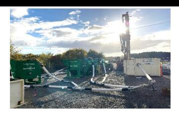
Experienced personnel were onsite, and they commenced test pumping on day two. Whilst test pumping the flow rate began to decrease from 30 l/s. The pump operatives sought to correct the drop in flow by increasing the frequency of the pump. Due to a build-up of pressure, one of the flexible pipes burst and water was released.
