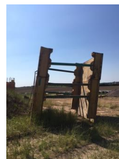
Photo 2: Trench box that was being lifted at time of incident
